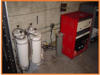
KA0FMZ repeater in Olathe, KS 147.240/151.4 MHz Repeater in red cabinet. 4 Large gray duplexers for 2m. Duplexers enable the use of 1 antenna for receive and transmit at the same time.
